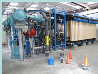
Pall Microfiltration Membrane 4 MGD
