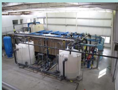
Pall Microfiltration Membrane 4 MGD
